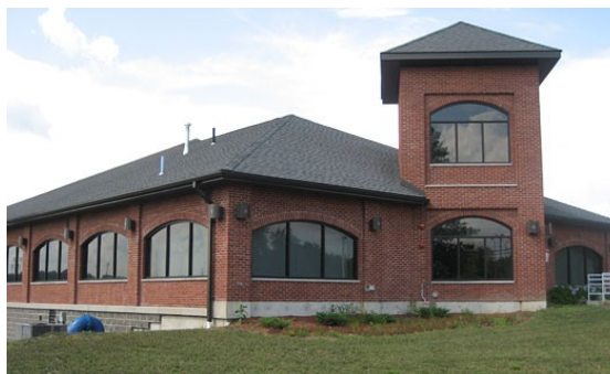
The Harold P. Naughton Water Filtration Facility
